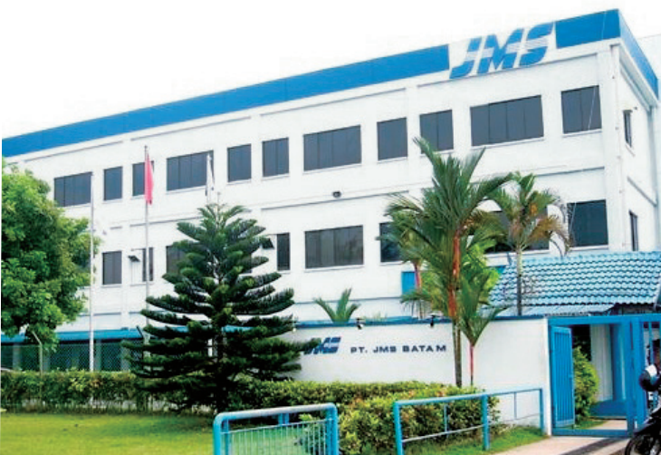
JMS Manufacturing Plant in Batam, Indonesia
